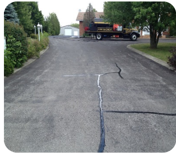
Crack Sealing
