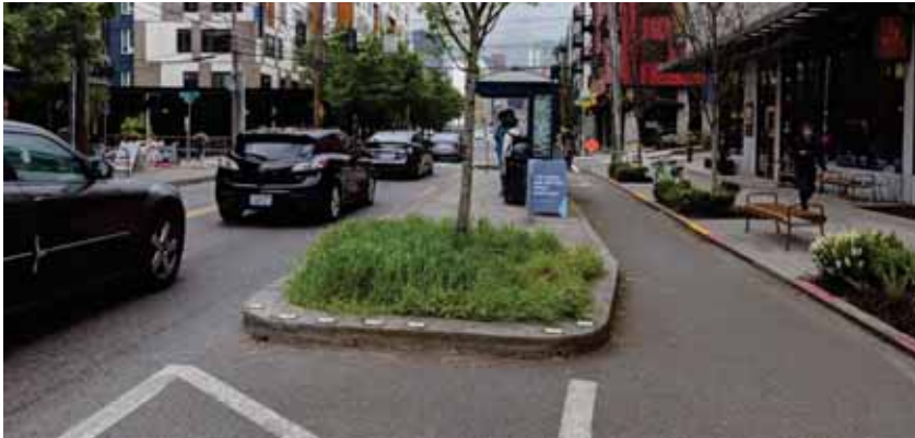
A transit side boarding island clarifies user spaces and minimizes conflict between bicyclists, pedestrians, transit passengers, buses, and vehicles.
