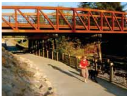
Shared Use Paths offer pedestrians and bicyclists space to be active away from vehicle traffic. Source: Peter Stetson.
