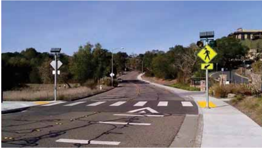
Raised pedestrian crossings help reduce vehicle speeds and give pedestrians greater prominence as they cross the street.
