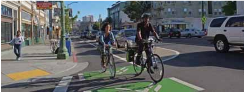
Parked cars serve as a barrier between bicyclists and the vehicle lane. Barriers could also include flexible posts, bollards, planters, or other design elements. Source: Bike East Bay
