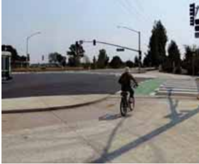
Protected intersections feature a corner safety island and intersection crossing markings.
