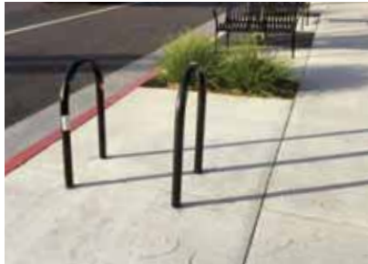
Inverted-U racks provide two points of contact.
