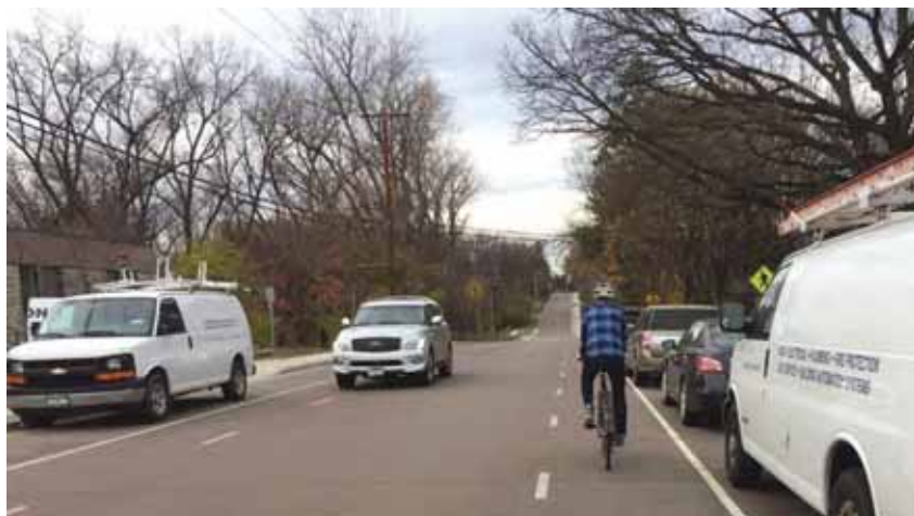
Advisory shoulders create usable shoulders for bicyclists on a roadway that is otherwise too narrow to accommodate one. The shoulder is delineated by pavement marking and optional pavement color. Motorists may only enter the shoulder when no bicyclists are present and must overtake these users with caution due to potential oncoming traffic.
